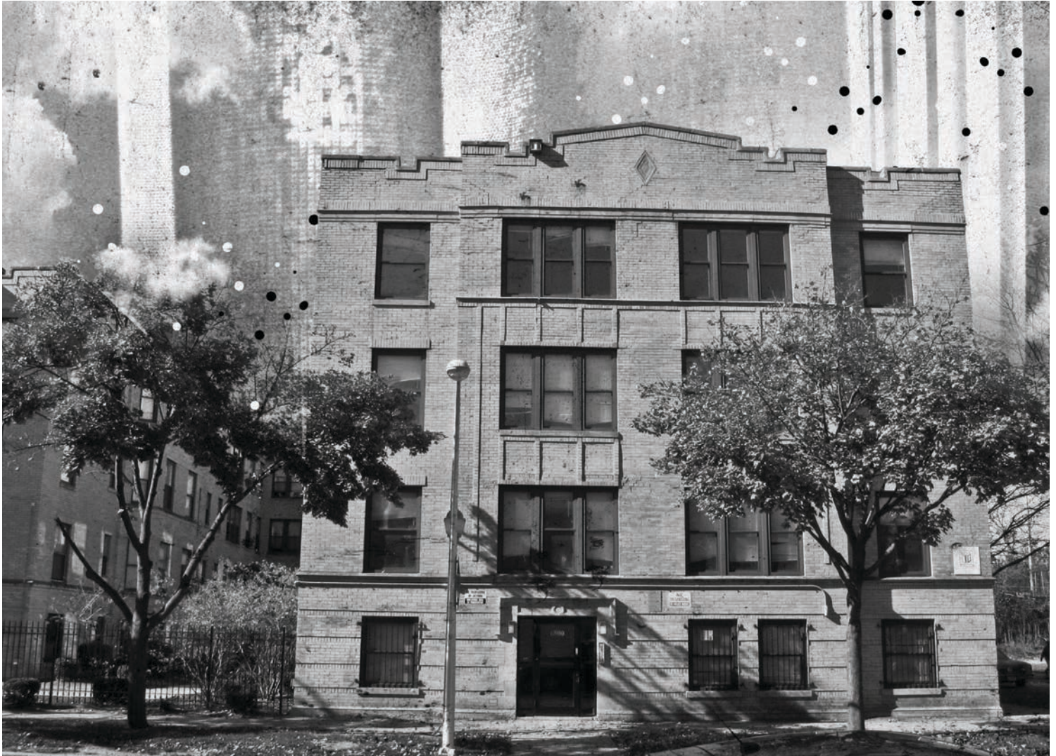
Chicago Low-Income Housing Trust Fund Rental Subsidy Program, Grand Crossing
