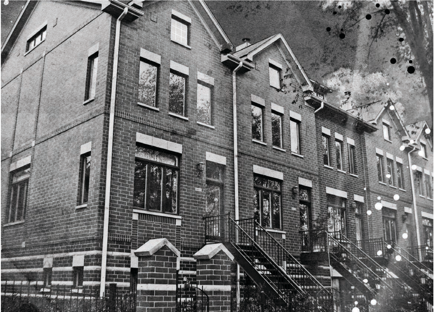
Affordable Requirements Ordinance, Ravenswood
